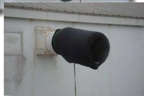
back-draft prevention equipment to prevent air from entering through idle exhaust fans.
